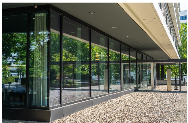
Image 3: The façade's original appearance was reproduced while meeting modern standards in terms of energy efficiency and statics. (Source: HUECK)
