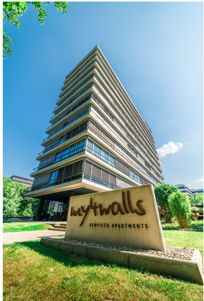
Image 1: In Hamburg’s “City Nord” area, the listed 1960s office building has been repurposed in line with modern thermal insulation and fire protection requirements. (Source: HUECK)
